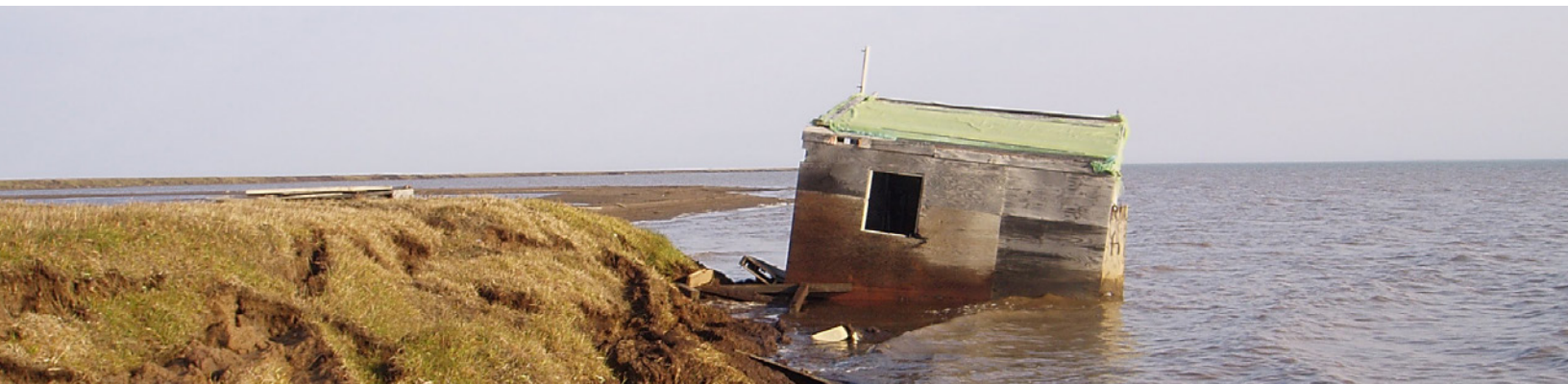
A cabin along Alaska's Arctic coast was washed into the ocean because the bluff it was sitting on eroded away. (Benjamin Jones/USGS)
