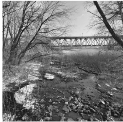
10. Restricted area under the bridge
