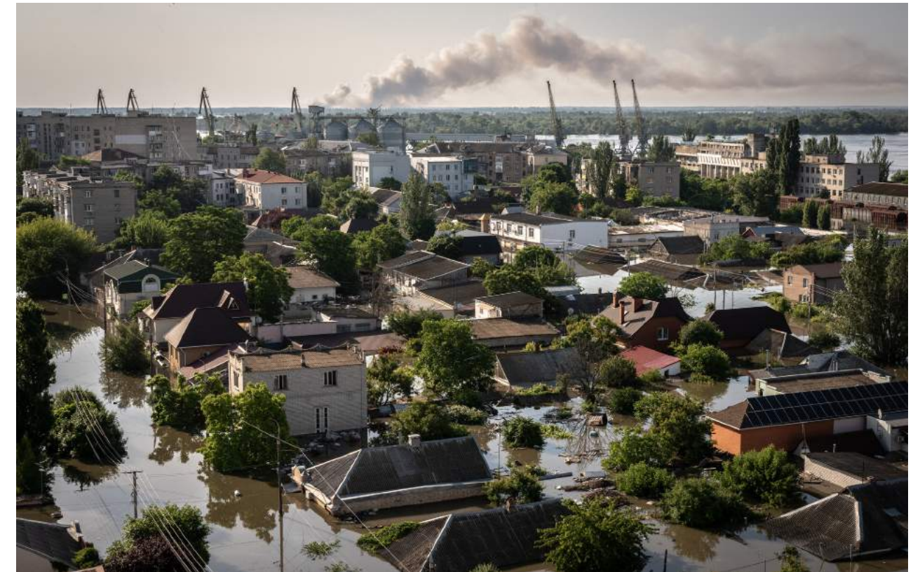
Figure 7. Photo of the city of Kherson flooded by the waters of the Dnipro River, after the destruction of the Kakhovka dam. Port cranes and grain elevators seen on the background have also been impacted. Author/Source: Alyona Budagovska.
