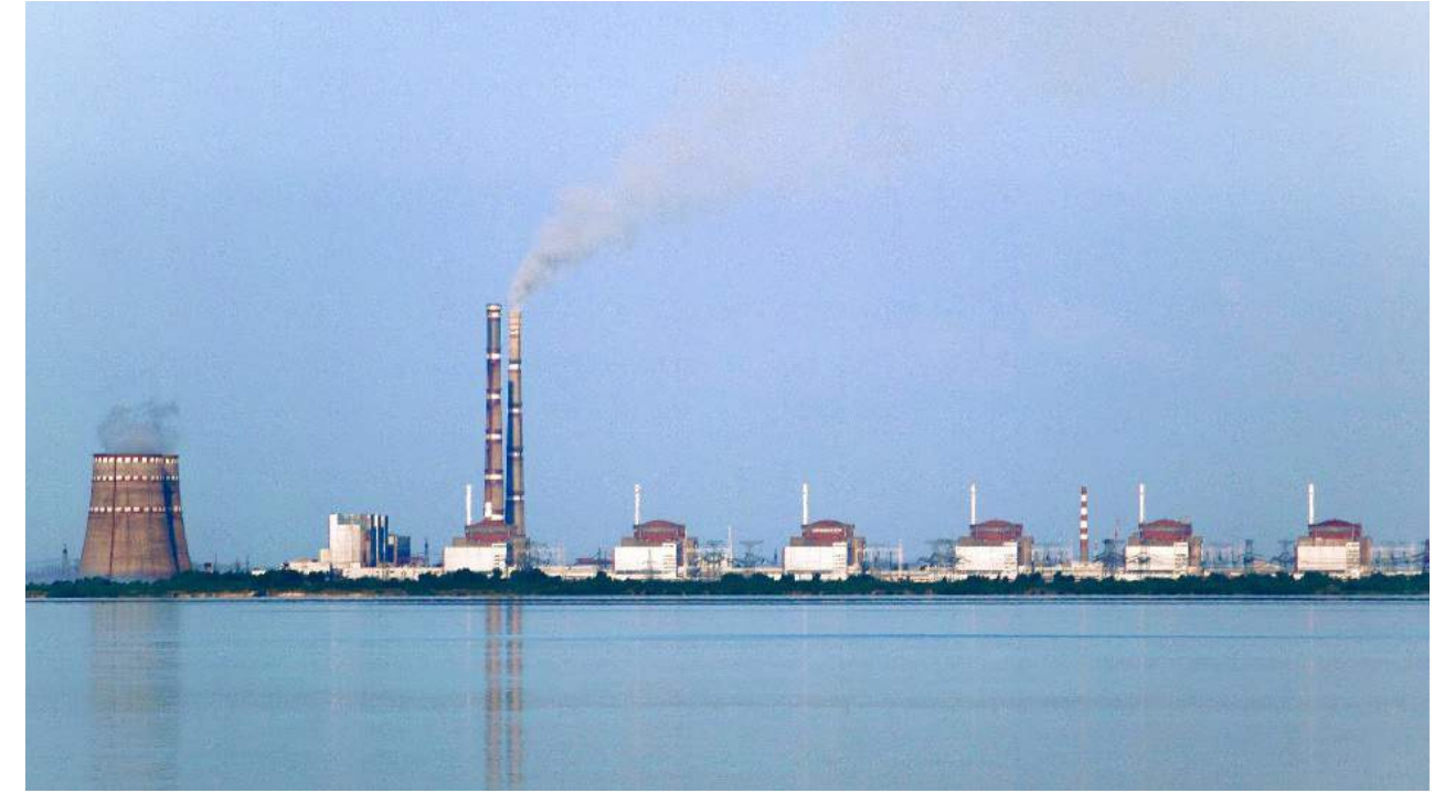
Figure 5. Photo of the Zaporizhzhia Nuclear Power Plant (2 cooling towers on the left and 6 VVER reactor buildings) and the Zaporizhzhia Thermal Power Plant (two tall smokestacks), viewed from across the Kakhovka Reservoir on the Dnipro River. Author: Ralf1969; Source: Wikipedia (Public Domain; CC BY-SA 3.0), 2009.
