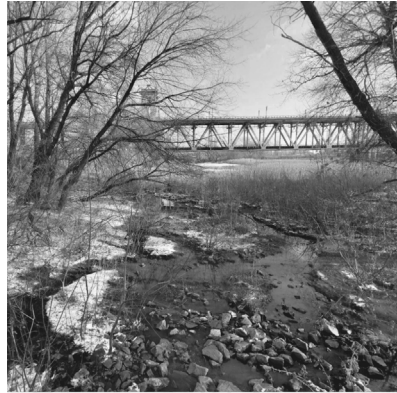
10. Restricted area under the bridge
