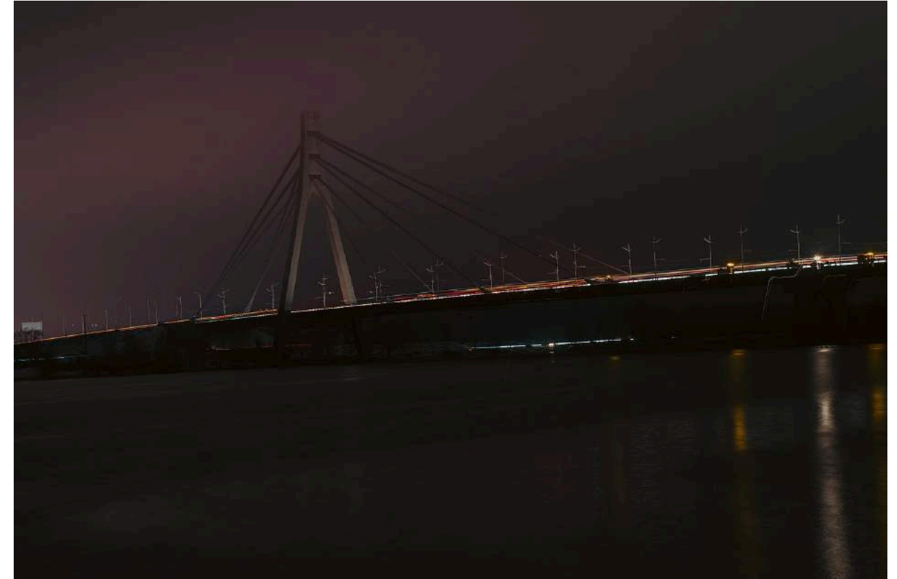
Figure 1. A photo of the Northern Birdge over the Dnipro River in Kyiv illuminated by car headlights during a "blackout", as the city is left without electricity supply after critical civil infrastructure was hit by Russian missile attacks, amid Russian military aggression of Ukraine, November 2022. Author: Valery Hitraya; Source: Wikipedia.org (CC BY-SA 4.0).
