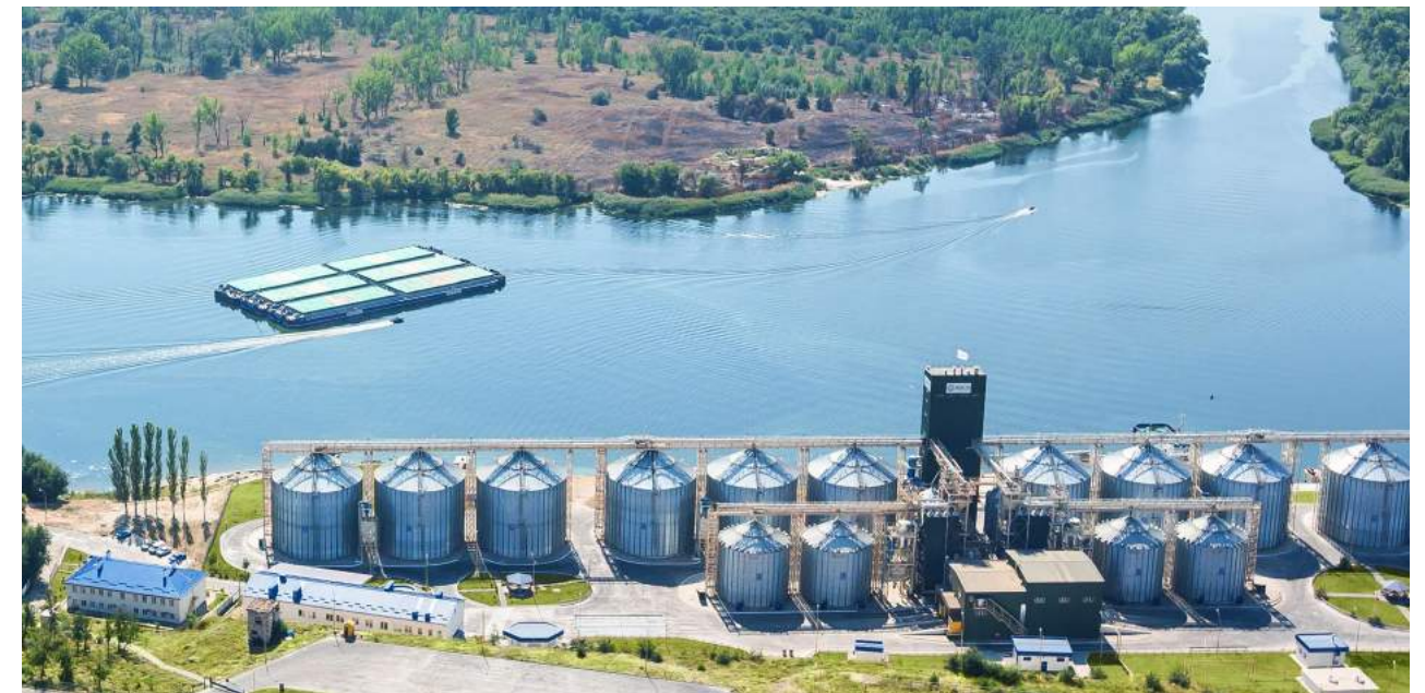
Figure 6: Photo of Nibulon's Terminal "Kozatska" (Kherson region). Commissioned in July 2012, it was designed for the storage and transshipment of grain and other agricultural cargo. In 2017, the storage capacities were expanded to 76,000 tons. In 2023, the branch was completely destroyed and flooded following the Russian destruction of the Kakhovka dam upstream. Author: unknown; Source: Nibulon, www.nibulon.com
