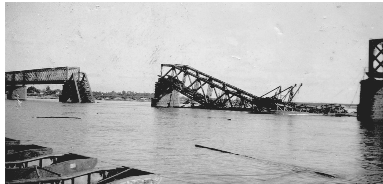
Figure 1. Bridge in Kremenchuk, 1941 Source: fund of the Kremenchuk Museum of Local Lore
