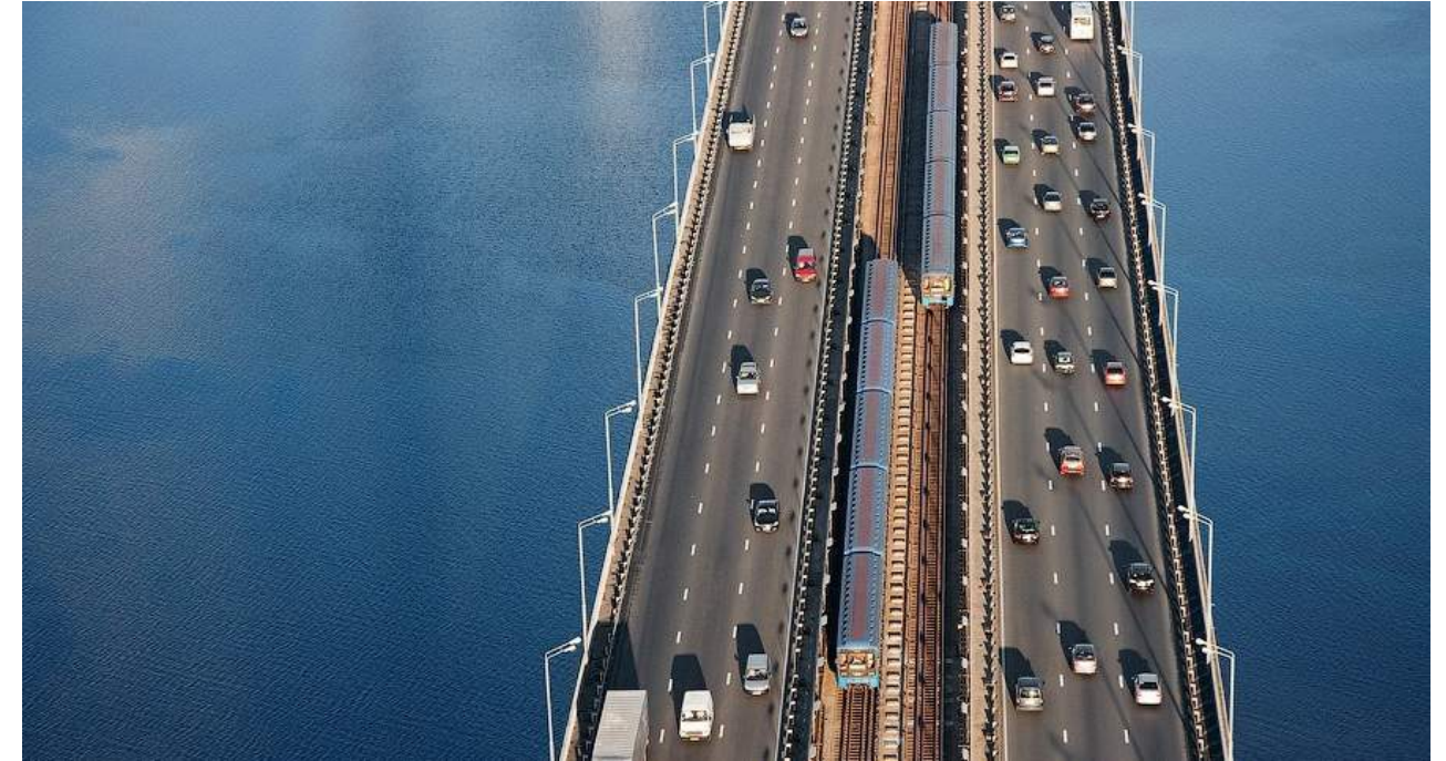
Figure 11: Photo of the Southern Bridge in Kyiv which both metro and automobile linkage Author: Oleg Totskiy ; Source: Wikipedia.org (CC BY-SA 3.0)
