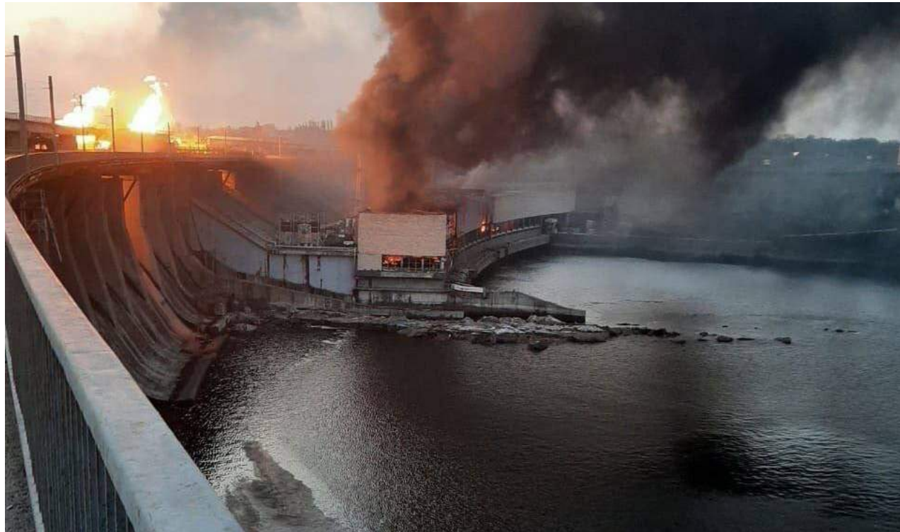
Figure 3. Photo of the damaged DniproHES, after a Russian missile and drone attack on March 22, 2024. Author: unknown; Source: Denys Shmyhal (Prime Minister of Ukraine) / Telegram
