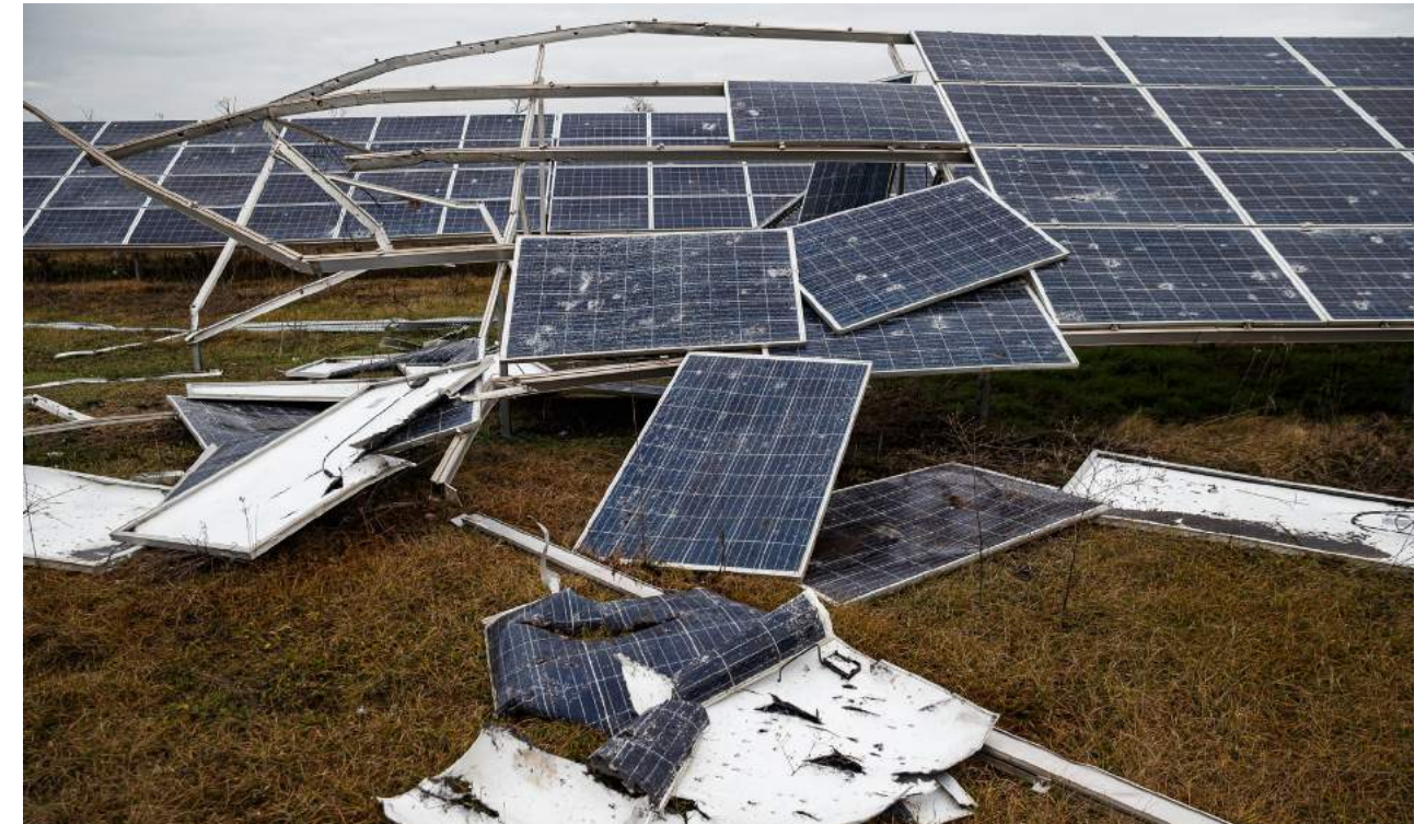
Figure 4. Photo of damaged photovoltaic panels as a result of Russian missile attacks. Author: unknown; Source: DTEK
