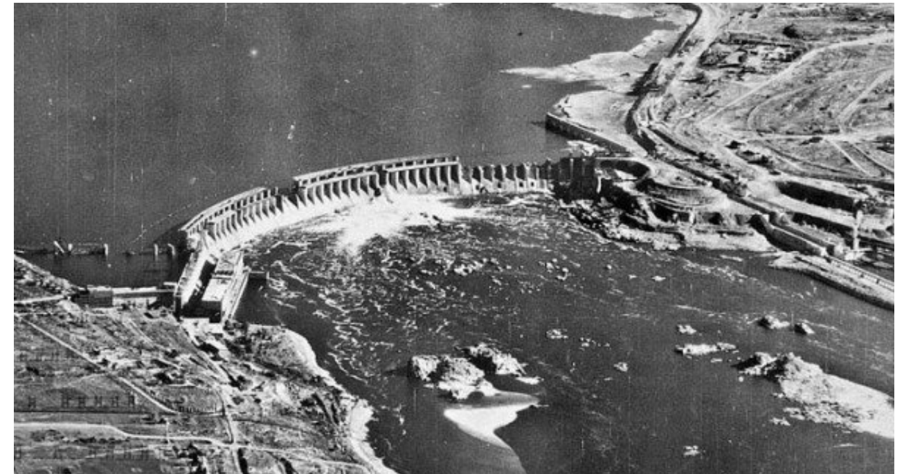
Figure 8. A german aerial photograph of the DniproHES in 1943, after the dam was again partly destroyed by the retreating Nazi German forces. Author: unknown; Source: Запорізький обласний краєзнавчий музей
