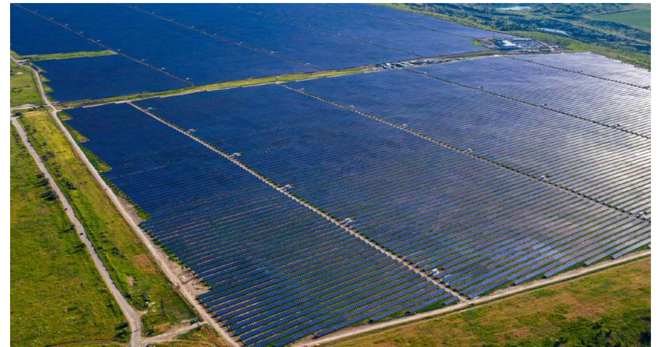
Figure 9: Photo of Nikopol Solar Power Plant (Dnipropetrovsk region) Author: unknown; Source: DTEK
