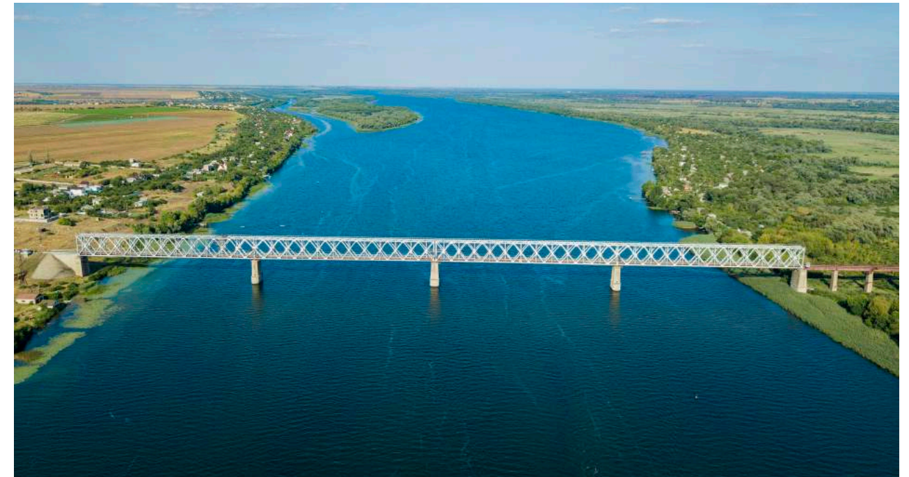
Figure 12: Photo of the Antonivsky Railway Bridge in the Kherson region, 2017 Author: Yevhenii Ihnatiev ; Source: Wikipedia (CC BY-SA 4.0)
