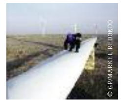
image A MAINTENANCE WORKER MARKS A BLADE OF A WINDMILL AT GUAZHOU WIND FARM NEAR YUMEN IN GANSU PROVINCE, CHINA.
