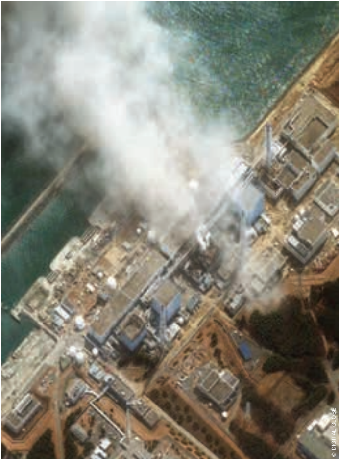
IMAGE SATELLITE IMAGE OF JAPAN'S DAI ICHI POWER PLANT SHOWING DAMAGE AFTER THE EARTHQUAKE AND TSUNAMI OF 2011.
