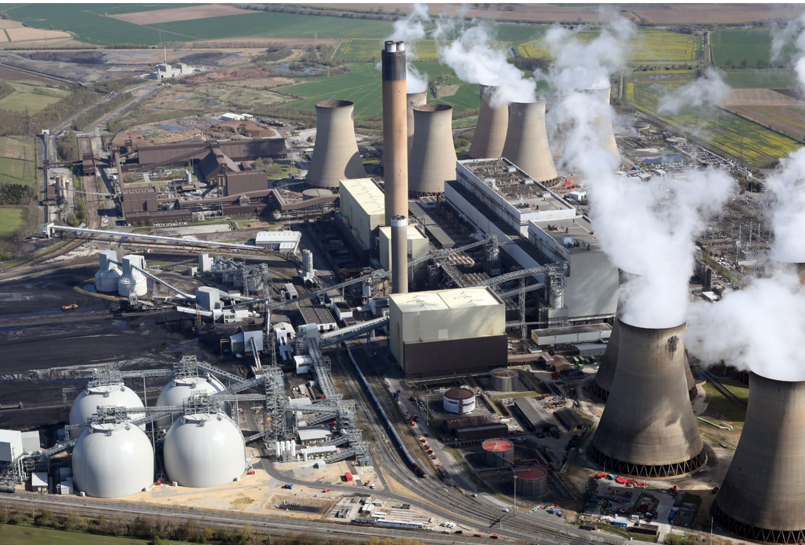
Drax, a 3960 MW coal-fired power station in North Yorkshire, England. It is the EU's third largest thermal power station by nameplate capacity and generates around 7% of UK's electricity. In 2012 the conversion to full biomass firing for three units was announced to be completed in 2013, 2014 and 2017 respectively. Photo © Neil Mitchell
