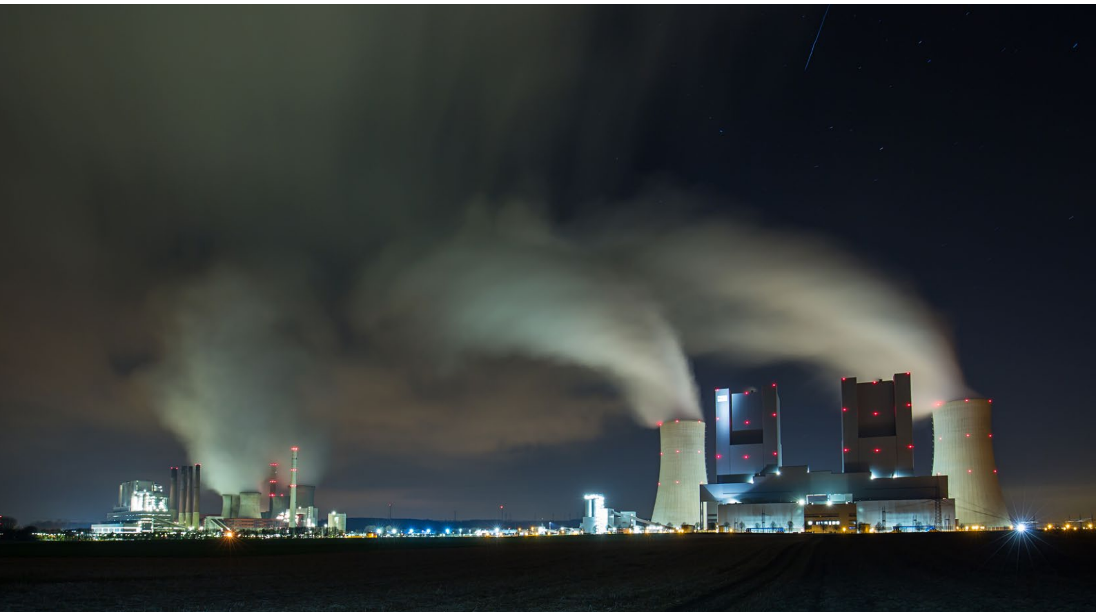
Kraftwerk Neurath at night. The 4400 MW lignite-fired power station in Neurath, North Rhine-Westphalia, Germany is the second largest in the EU. The five units on the left were built in the 1970's and the two 1100 MW units on the right were completed in 2012. Photo © r.classen
