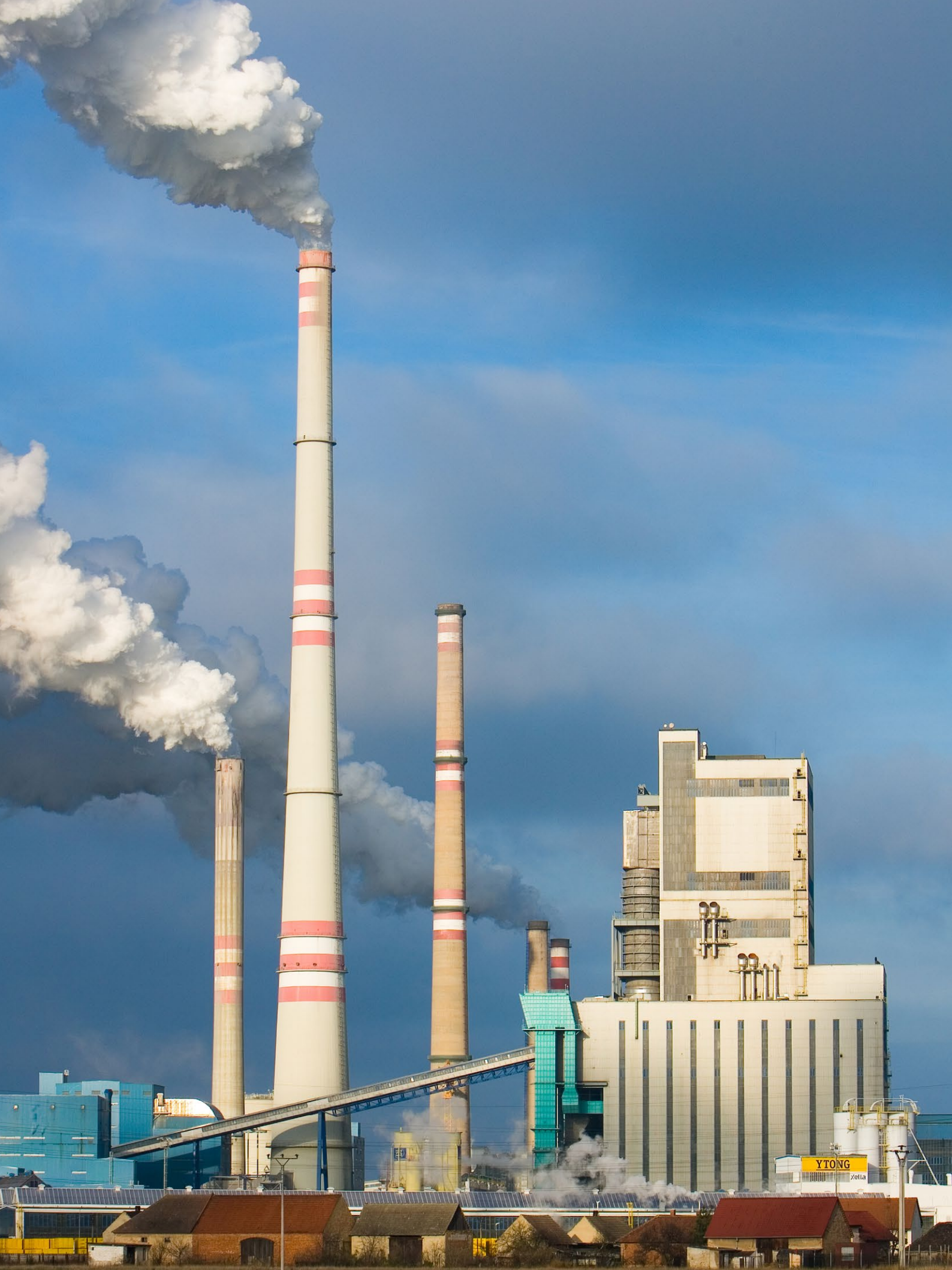
The Melnik Power Station in the Czech Republic. The 1050 MW four unit plant is fueled by lignite from mines in North and West Bohemia. Photo © BESTWEB
