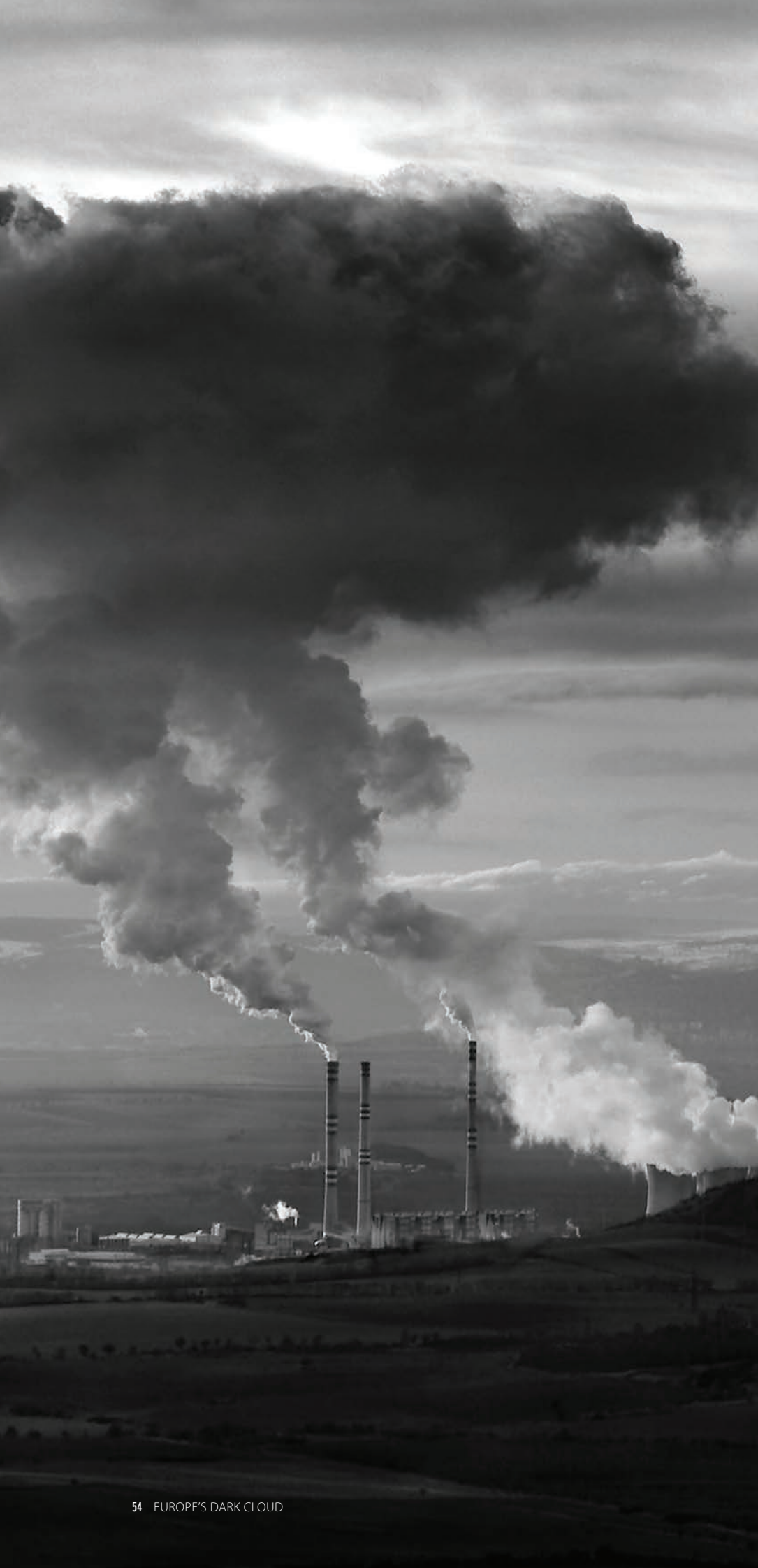
POČERADY POWER PLANT, CZECH REPUBLIC. © zahorec
