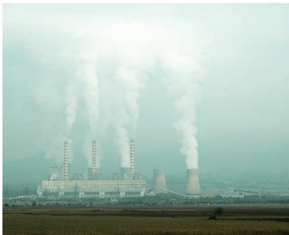
AGRIOS DIMITRIOS POWER PLANT. © Ioannis Tokaris
