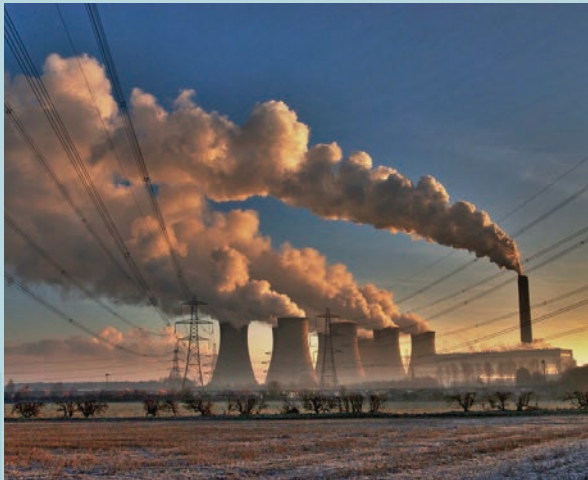
EGGBOROUGH POWER PLANT. © John Mabbitt
