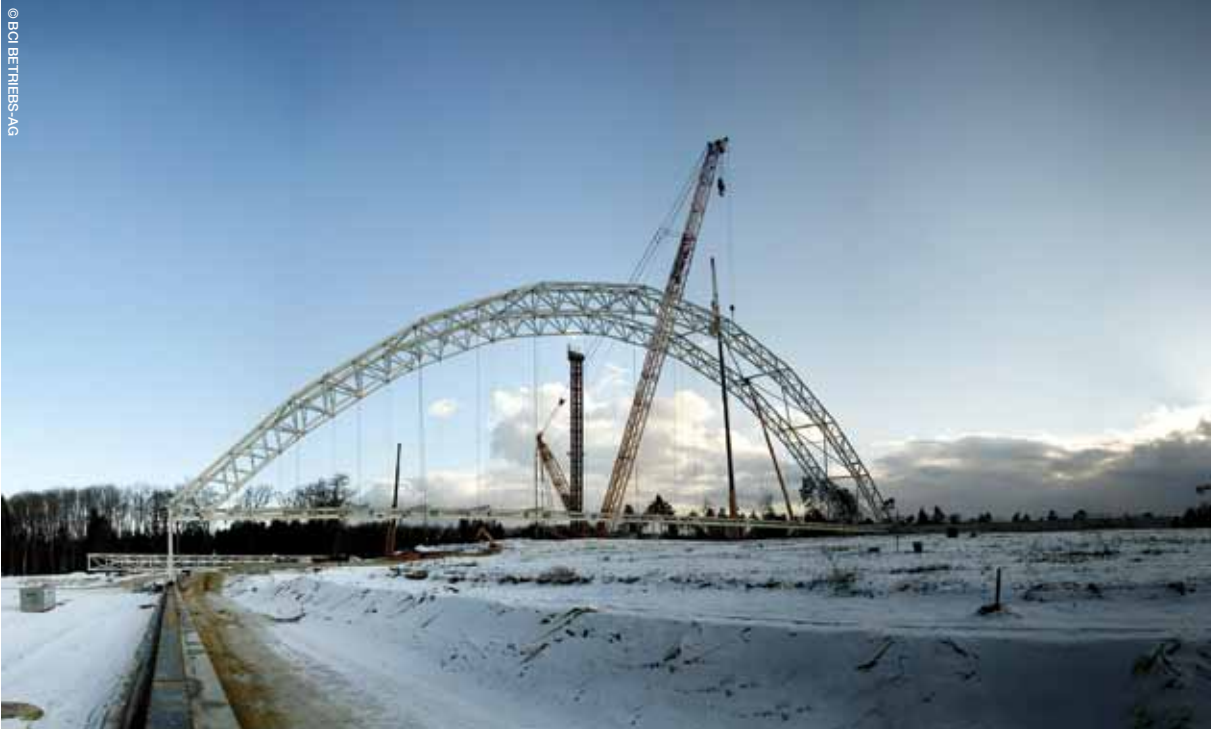
image: Construction of the clean-up hall at Bonfol
