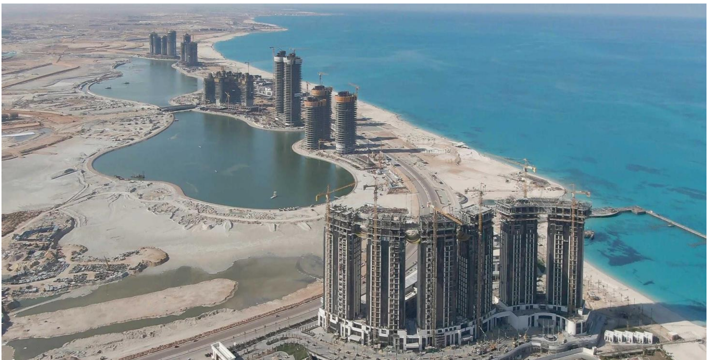
Construction of towers in New Alamein City
