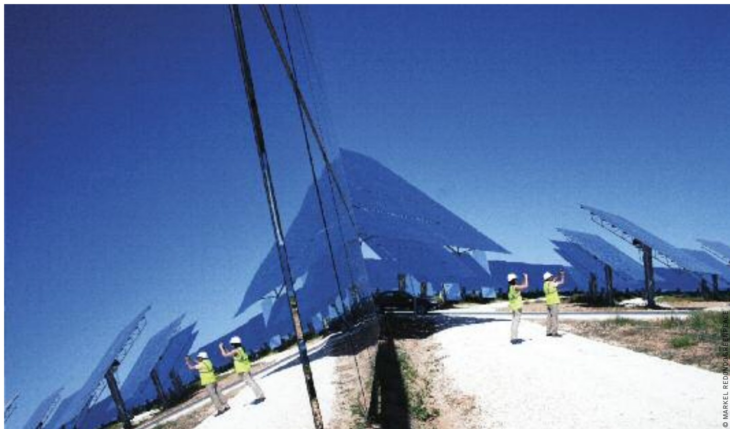
image GEMASOLAR, A 15 MWE SOLAR-ONLY POWER TOWER PLANT. ITS 16-HOUR MOLTEN SALT STORAGE SYSTEM CAN DELIVER POWER AROUND THE CLOCK.
