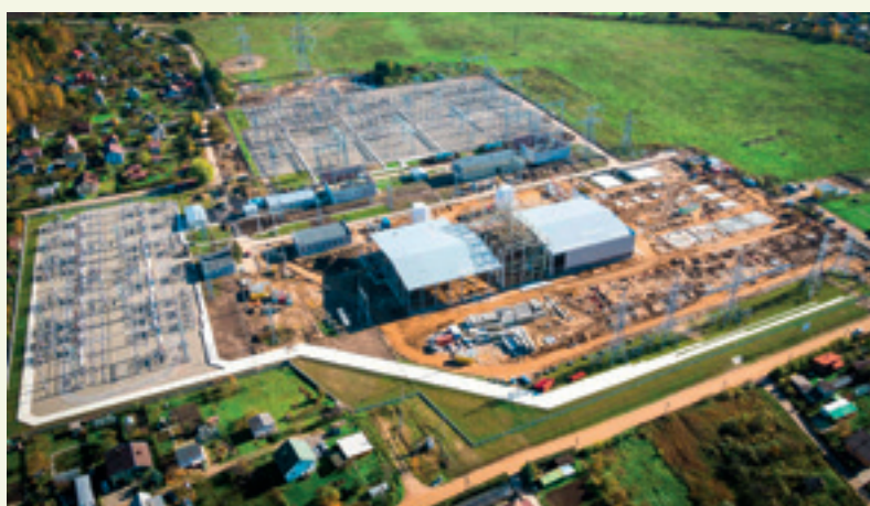
Photo 3 — NordBalt ground station in Klaipeda, Lithuania
