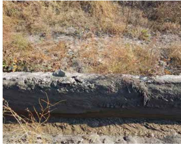
Figure 10. Solid material built up on the sides of the concrete channel used to transport ash slurry, close to the Kamenik ash disposal site
