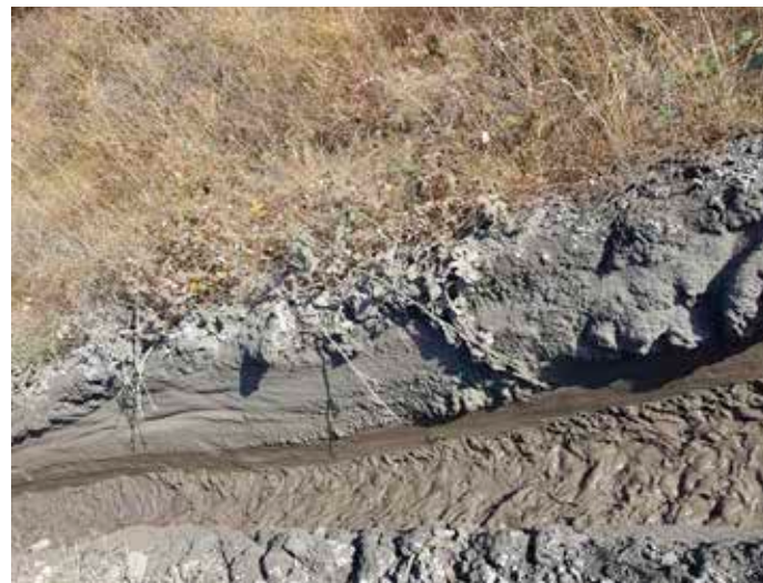
Figure 10. Solid material built up on the sides of the concrete channel used to transport ash slurry, close to the Kamenik ash disposal site
