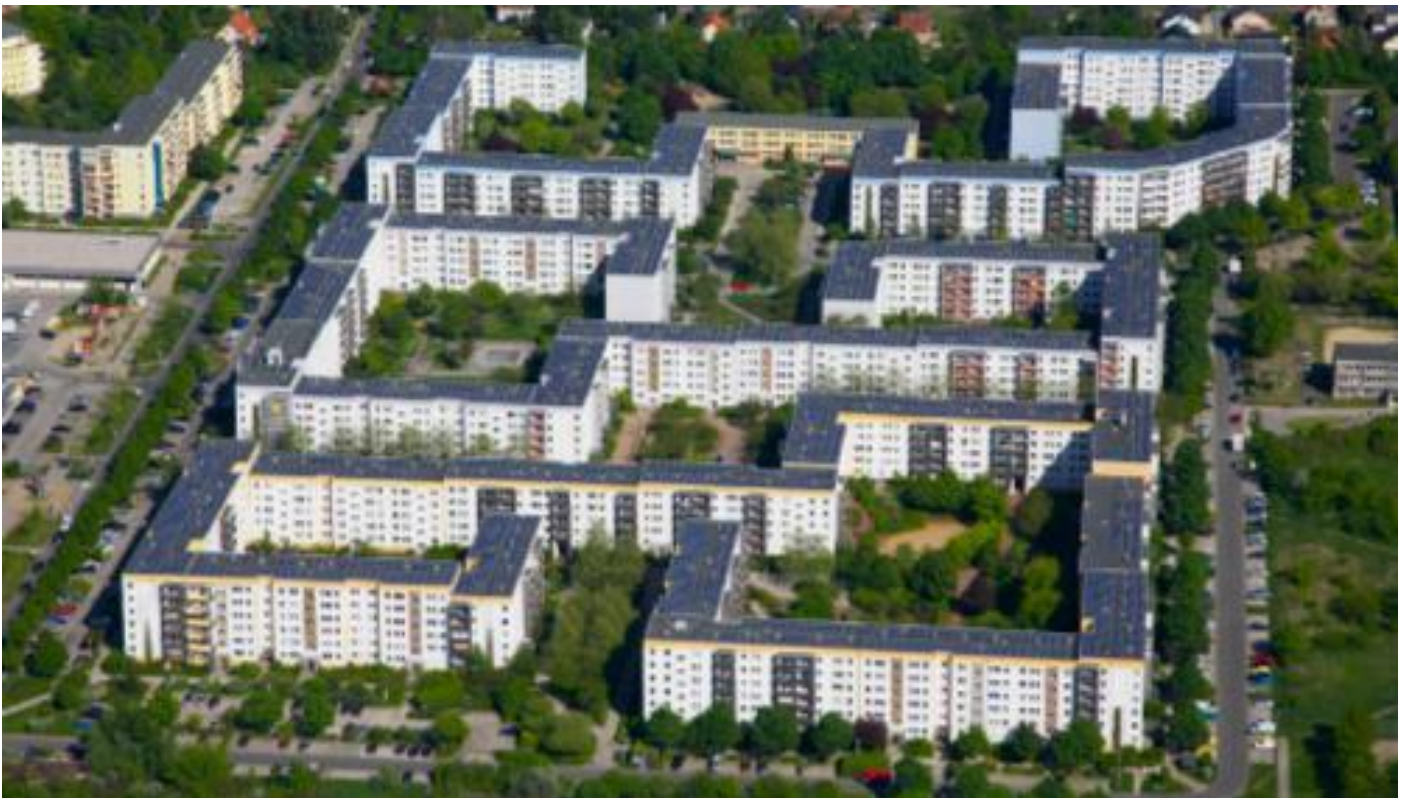
Photovoltaic panels on rooftops of rehabilitated concrete blocks of flats in East Berlin; Gelbe Viertel project by LichtBlick; Photo: LichtBlick
