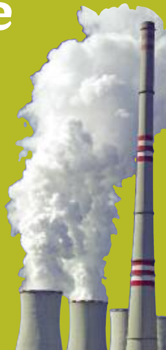
image COAL FIRED POWER PLANT. © F. FUXA/DREAMSTIME
