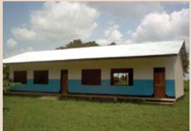
2 classrooms built at Mbasa primary school. © Oakland Institute
