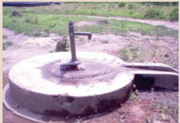
Manual pump well built at Mbasa primary school. © Oakland Institute
