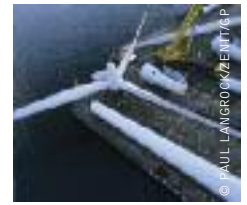
image CONSTRUCTION OF THE OFFSHORE WINDFARM AT MIDDELGRUNDEN NEAR COPENHAGEN, DENMARK.
