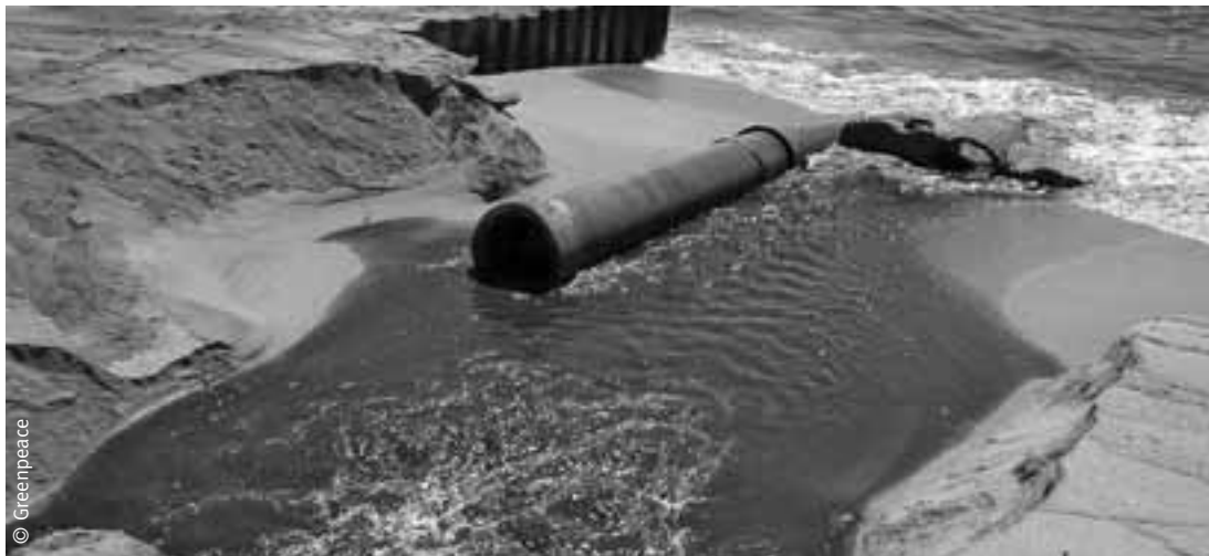
Abocament contaminant a Pineda de Mar, Barcelona.
