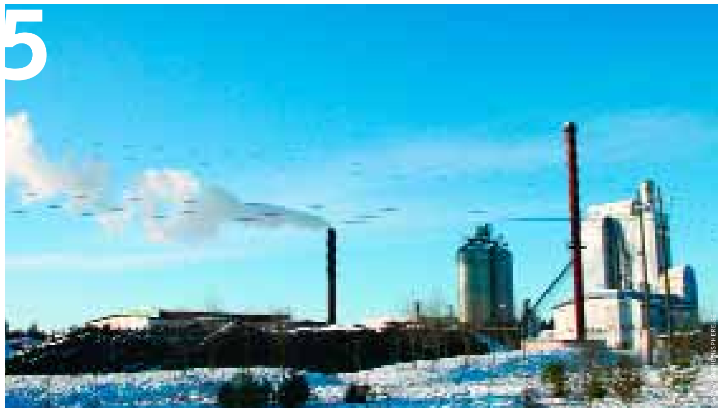
image BIOMASS ENERGY PLANT NEAR VARNAMO, SWEDEN.
