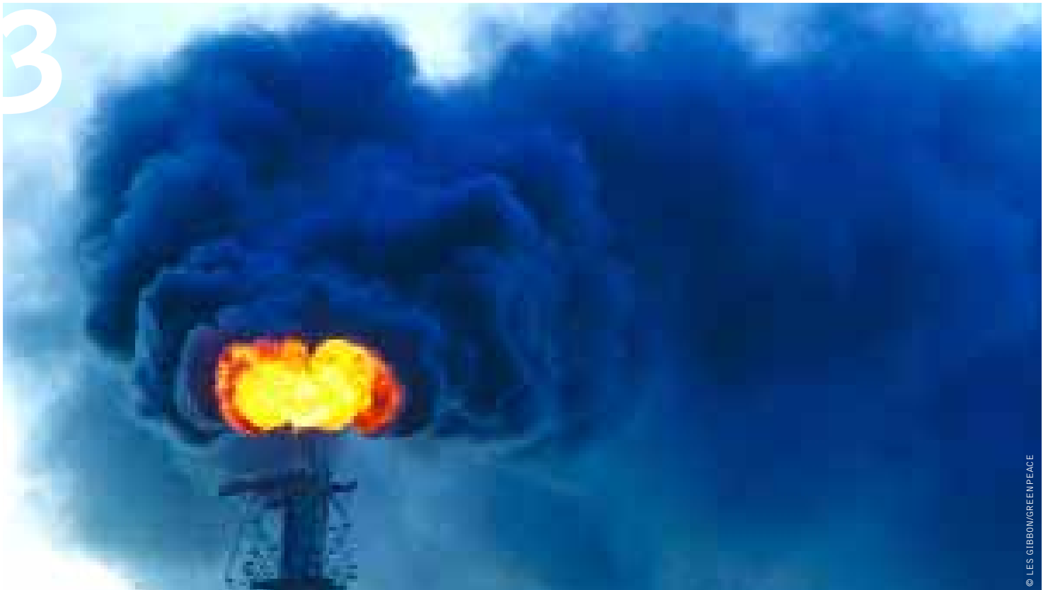
image FLARE STACK AT AN OIL REFINERY IN IMMINGHAM, UK.
